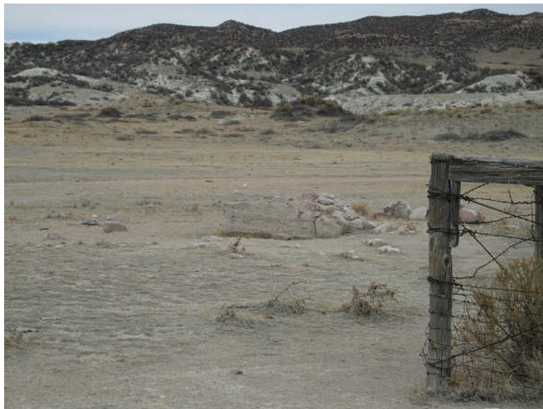
Soapstone School foundation
